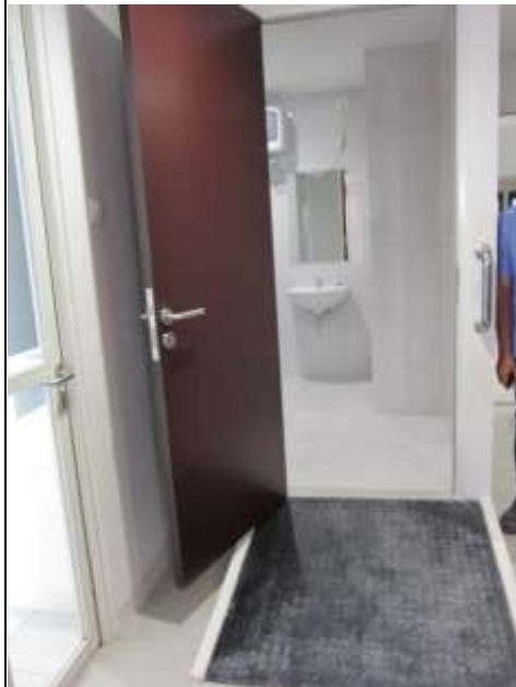
Ramp to accessible bathroom
